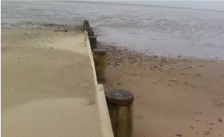
Figure 5 – Groynes, an example of coastal management
